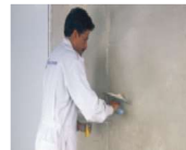
Step-4 Thin slurry coat for finishing
