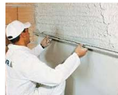
Step-3 Flatten the Plaster
