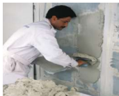
Step-2 Filling plaster material
