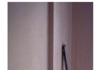
Step-6 Ready surface for painting
